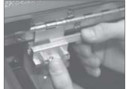
Pictured: Attaching Hinge Bracket to Cover.
