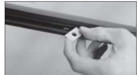
Insert the support washers (D) into the wind seal rails as pictured above.
