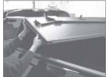
Pictured: Unfolding cover between wind seal rails.
